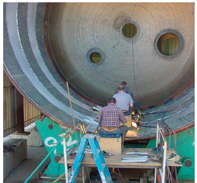
Homogeneous lead lining on site
