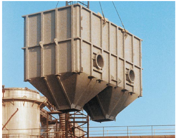
Installation of a complete wet electrostatic precipitator housing
